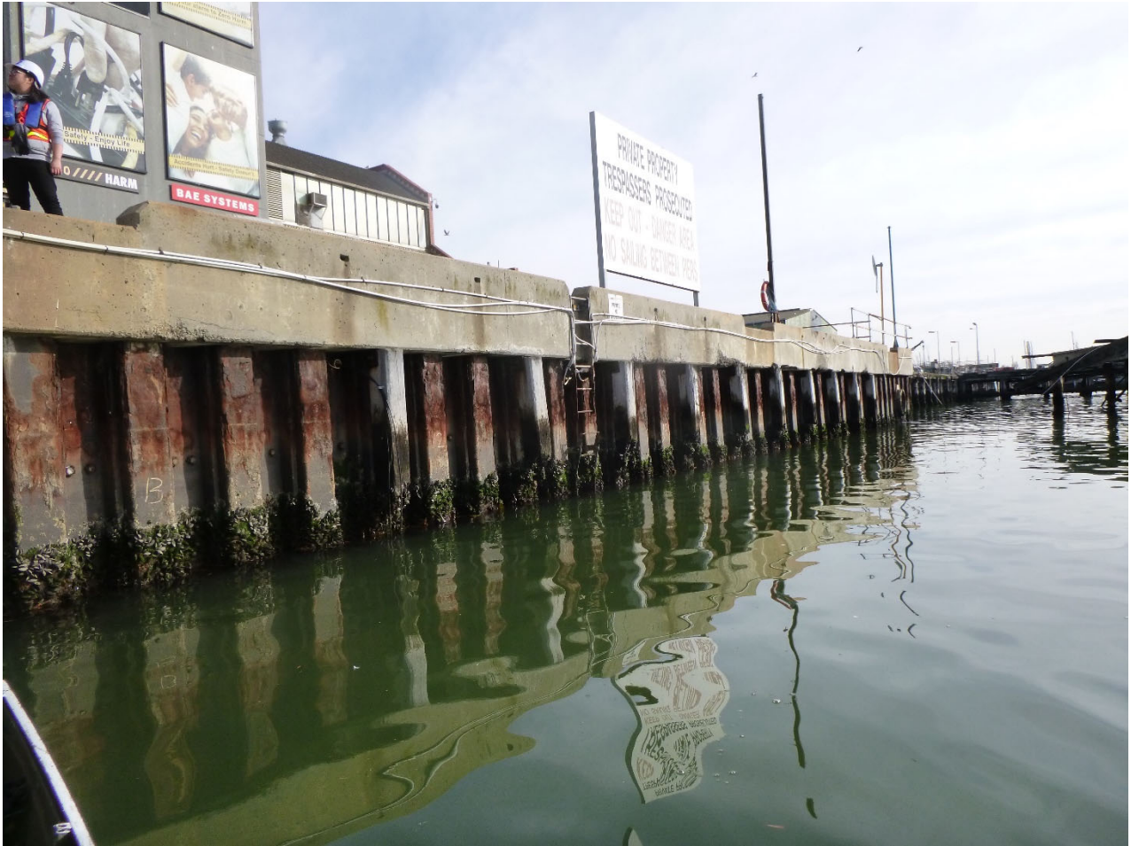
East end of Reid Pier at Williamstown, Victoria. Testing in 2018.
