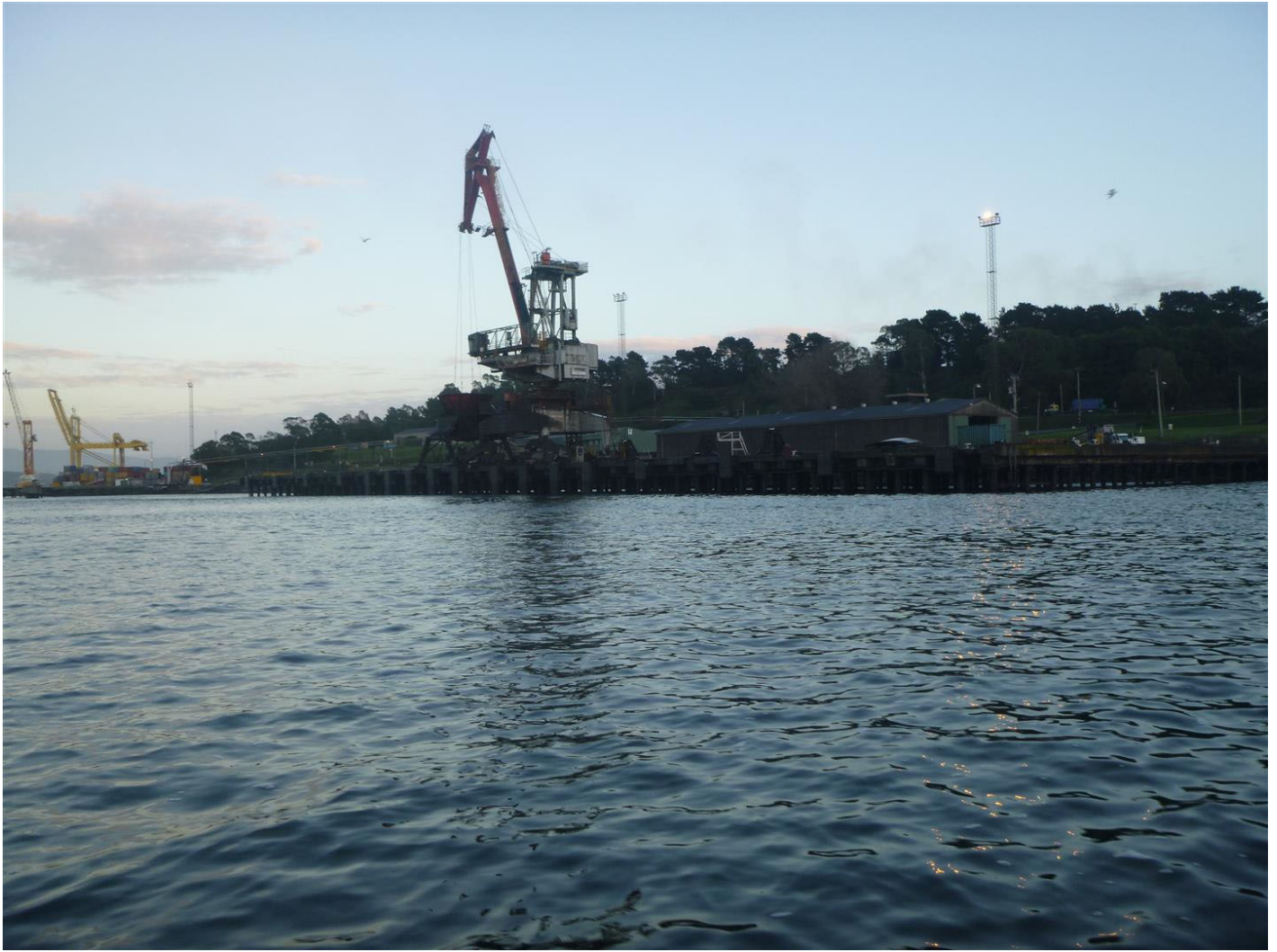
Bell Bay wharf, Tasmania, photos from the 2018 inspection and testing.
